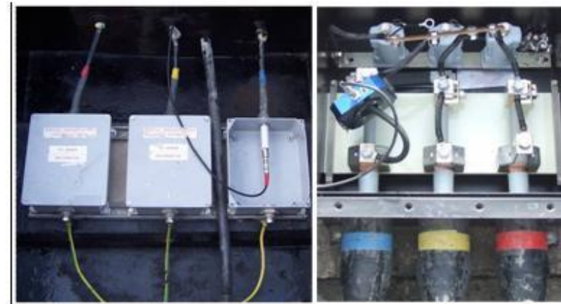
Sensors connection at link boxes
