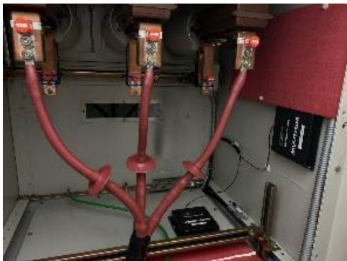
Switchgear Cable / Breaker Arm
