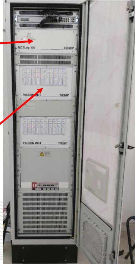
CMD Panel for switchboard located in S/S
